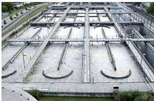
Wastewater, Sewage Treatment
